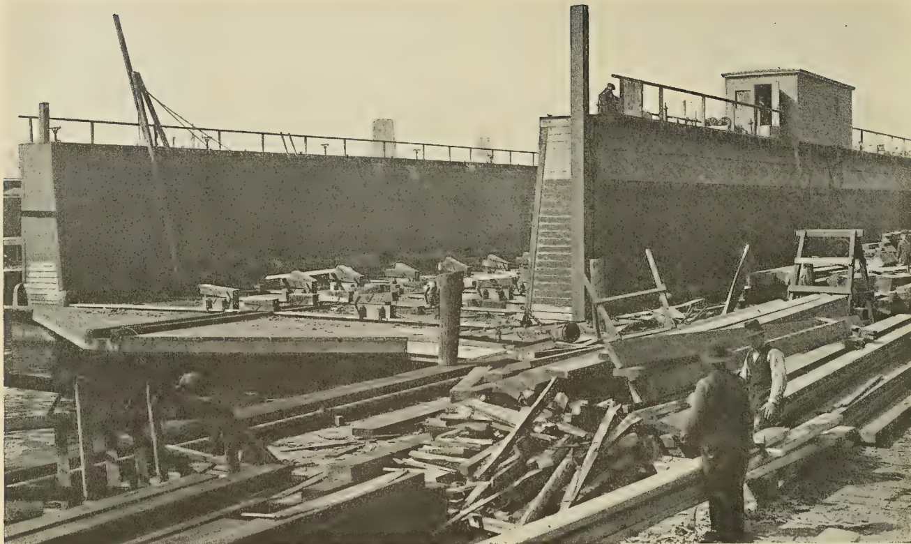
Fig. 1.—2,400-Ton Dock of Vulcan Iron Works, Under Construction
